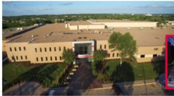
Lincoln, Nebraska Sending Plant
