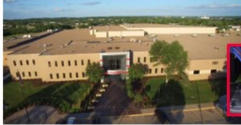
Lincoln, Nebraska Sending Plant
