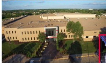
Lincoln, Nebraska Sending Plant
